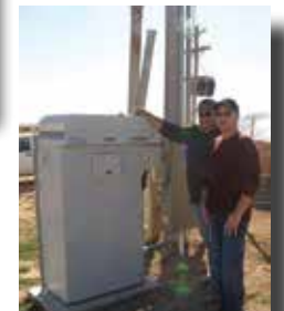
VFD installed on irrigation system.
