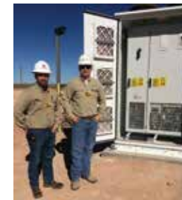
VFD installed in oilfield
